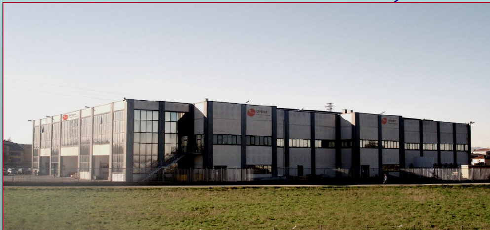
Orton factory and office's building
